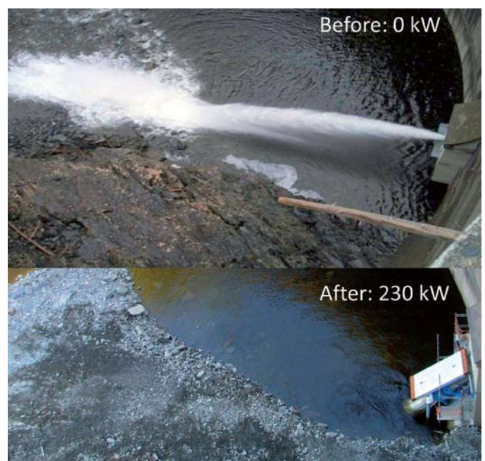
Reserved flow from Hegset dam before and after Turbinator installation
